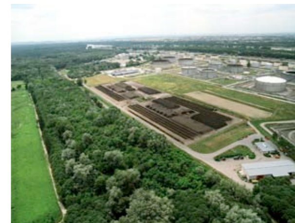
KOMPOSTWERK LOBAU der MA 48 COMPOSTING FACILITY of the municipal department 48
